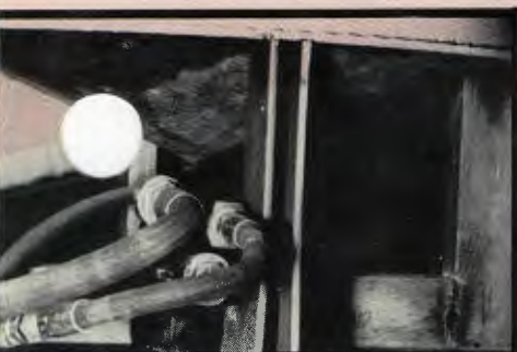
funnel construction, filter, lines and stand.
